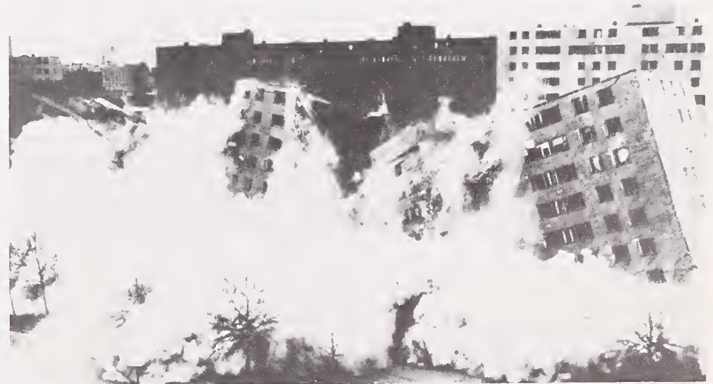
Pruitt Igoe—After (HUD)
